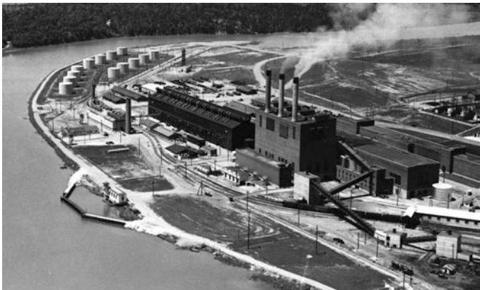
Fig. 5.28 The S-50 facility. The main process plant is the long, dark building to the left of center. The K-25 powerhouse (three smokestacks) is to its right, and a tank farm for supplying oil for the “new boiler plant” is to the left. The new boiler plant itself is between the main process building and the river. Source http://commons.wikimedia.org/wiki/File:S50plant.jpg
