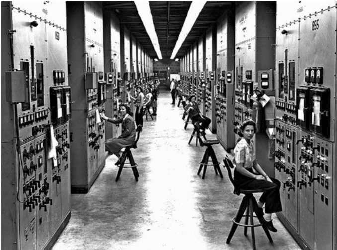
Fig. 5.17 “Calutron girls” at their operating stations. Each operator monitored the performance of two vacuum tanks, but had no idea what was being produced. Source http://commons.wikimedia.org/wiki/File:Y12_Calutron_Operators.jpg
