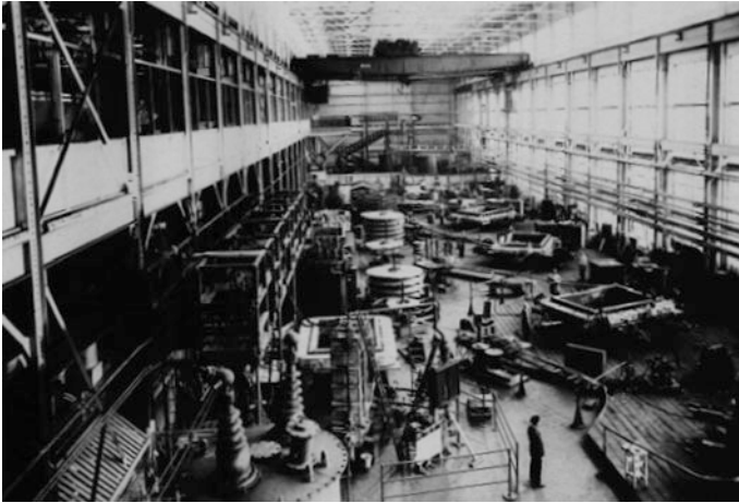
Fig. 5.21 This somewhat low-quality photograph, reproduced from a Manhattan District History microfilm, shows magnet coils being wound onto square bobbins, likely Alpha I coils. Note person in lower right foreground for scale. Source A1218(10), image 0443
