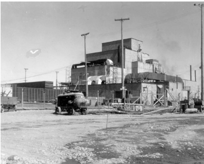
Fig. 6.4 The B-pile building under construction (HAER, Photo 3)
