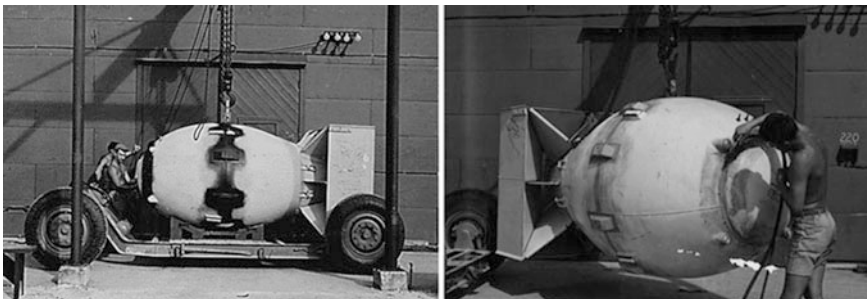
Fig. 7.16 Left: Assembled Fat Man bomb. Note signatures on tail. Sources http://commons.wikimedia.org/wiki/File:Fat_Man_on_Trailer.jpg . Right: On Tinian island, Fat Man receives a coat of sealant. Note FM stencil on nose. Source http://commons.wikimedia.org/wiki/File:Fat_Man_on_Tinian.jpg
