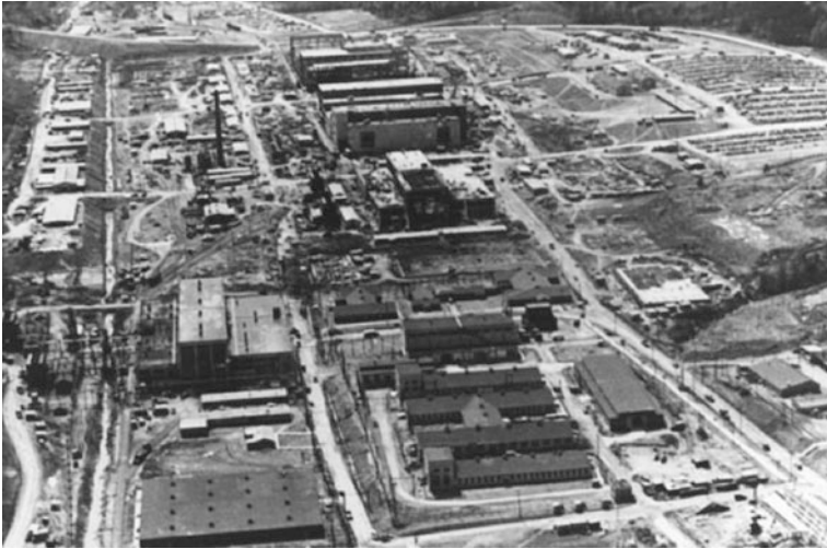
Fig. 5.22 Construction at Y-12, 1944. Source http://cdm16107.contentdm.oclc.org/cdm/search/collection/p15388cdi
